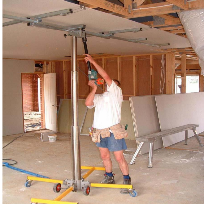
Pictured: a pneumatically-powered plaster sheet lifter with large extension screw gun
